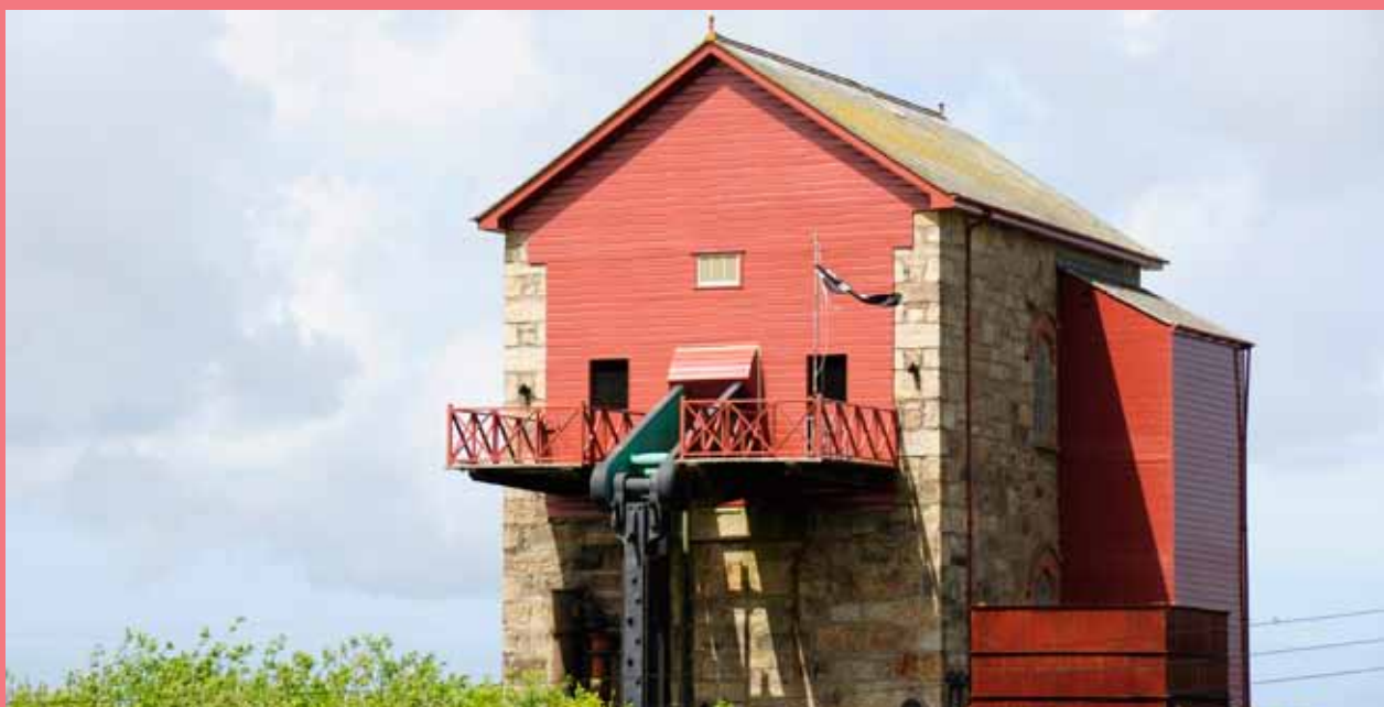
Above: The Taylor’s Shaft pumping engine at East Pool Mine, Pool
