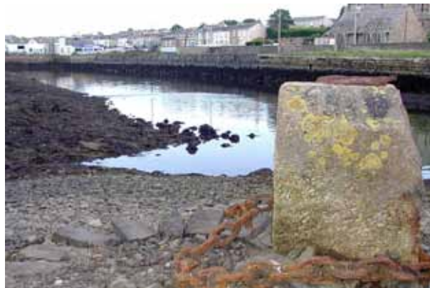
Above: Copperhouse Canal
