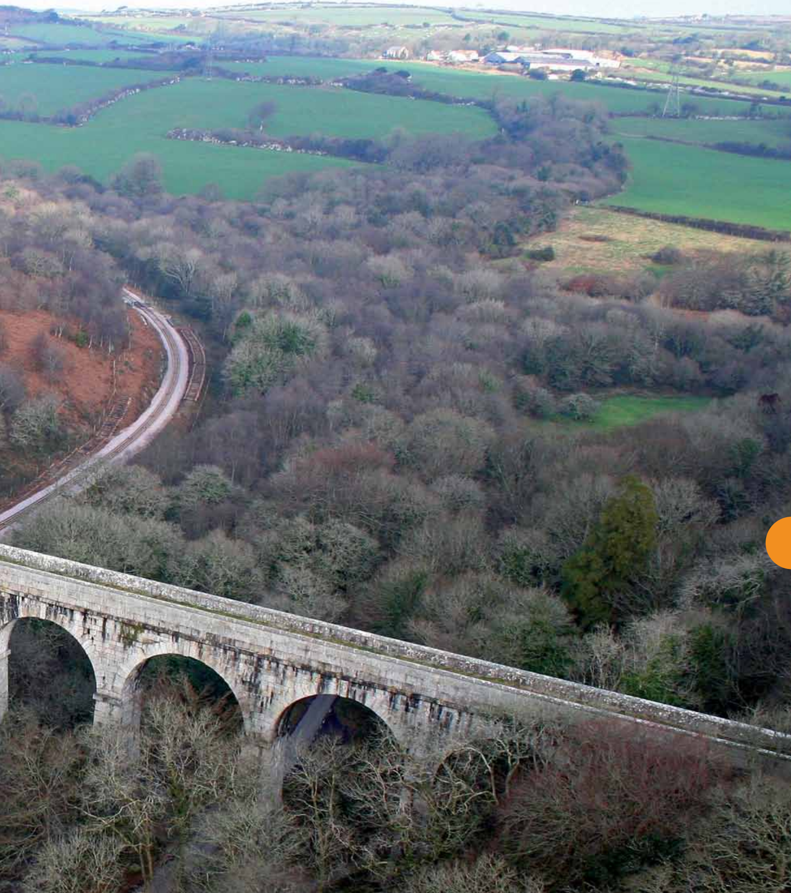
Above: The Treffry viaduct and aqueduct in the Luxulyan Valley
