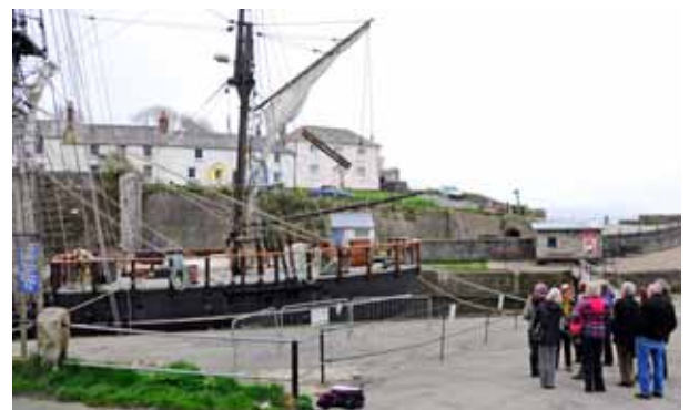
Above: Tourism businesses visiting the harbour at Charlestown on a World Heritage Site Familiarisation Day
