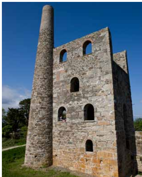
Above: the conserved pumping engine house at Wheal Peevor near Redruth
