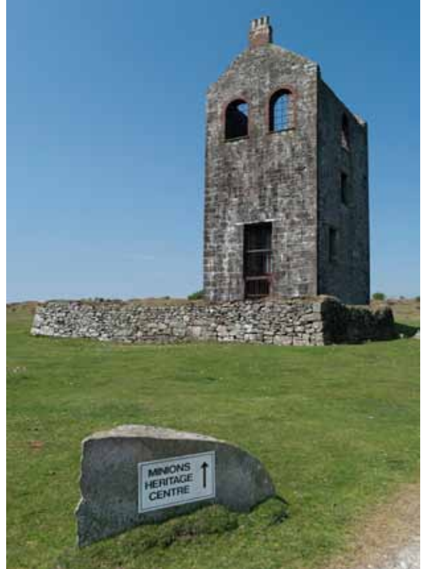
Above: The Minions Heritage Centre at Houseman's Shaft engine house, South Phoenix Mine
