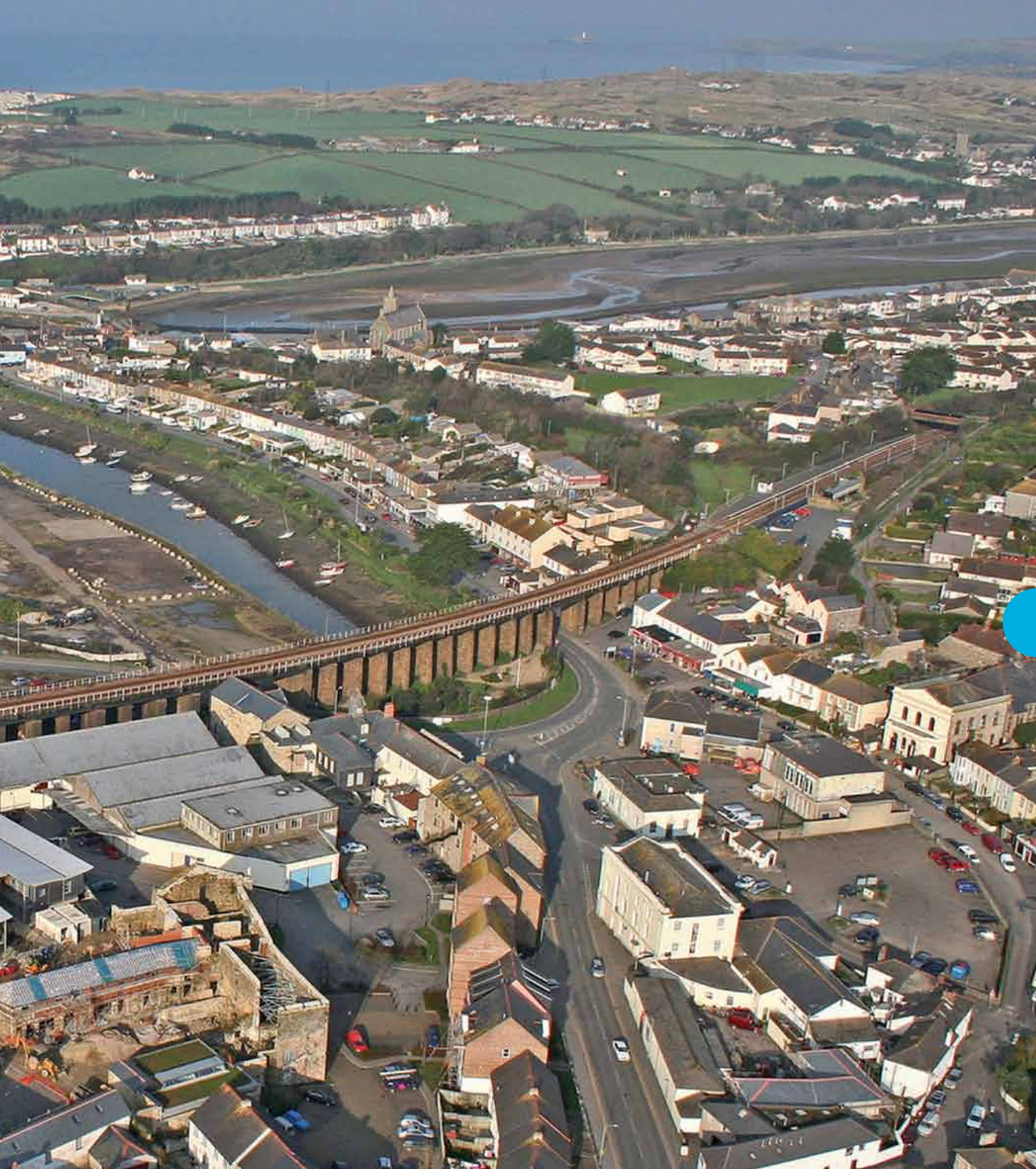
Above: Extensive harbour quays built to serve the foundry of Harvey & Co., Hayle, and what was once the world's greatest manufactory of the Cornish steam beam engine
