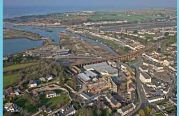
Above: Hayle and Harvey's Foundry
