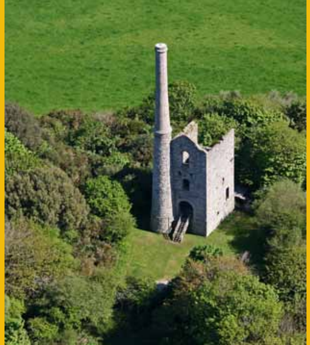
Above: Killifreth Mine – Hawke's Shaft Engine House
