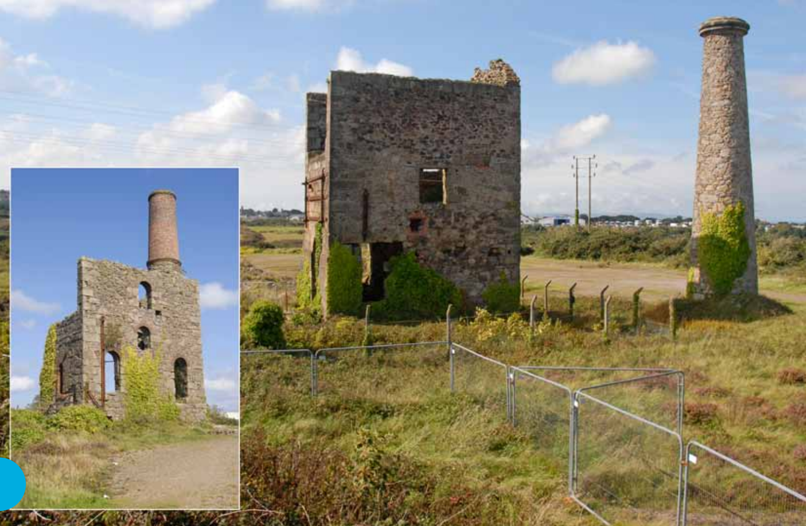
Above: Cooks Kitchen Mine, Pool
