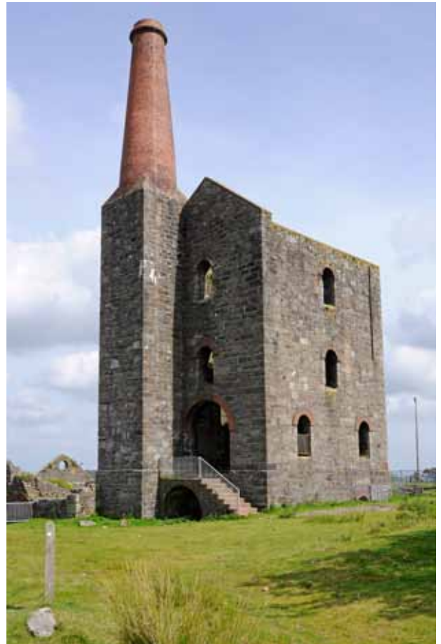
Above: The Prince of Wales Shaft engine house at Phoenix United Mine
