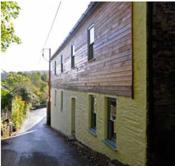
Top and above: The former Miner's Barracks of New Consols Mine Lockett, before and after conversion to a dwelling; note loss of original doorway, bottom centre-right
