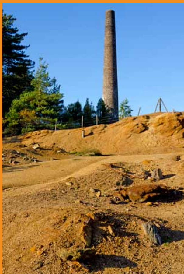
Above: Arsenic chimney at Devon Great Consols Mine
